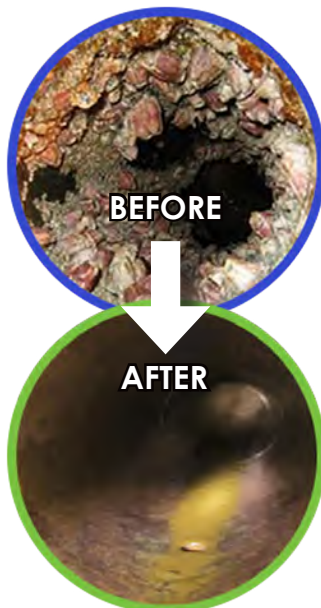
Water Piping Scale
