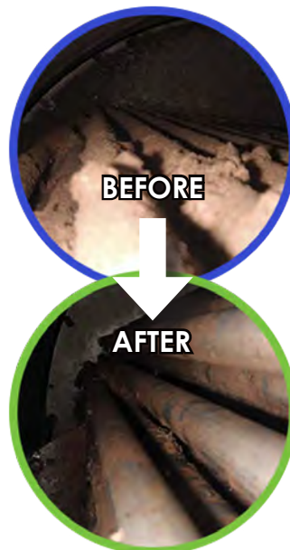
Heat Exchanger Scale
